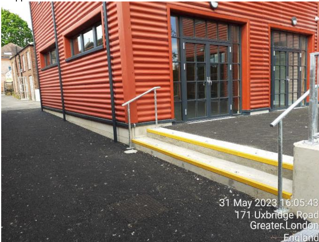
Stepped access to terrace:
